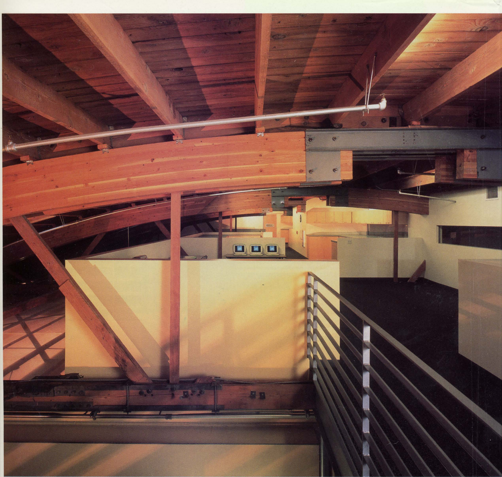
A mezzanine of study spaces and administrative areas are carved into the belly of the bow-string trusses (above), with operable skylights for improved ventilation. Larger double-height spaces include art studios and a music room (opposite, left and middle). The great hall ends with a student gallery and lounge wrapping offices and classrooms with translucent partitions for improved lighting (opposite, right). Throughout the spaces, the exposed construction offers a dynamic and textured backdrop for students.
