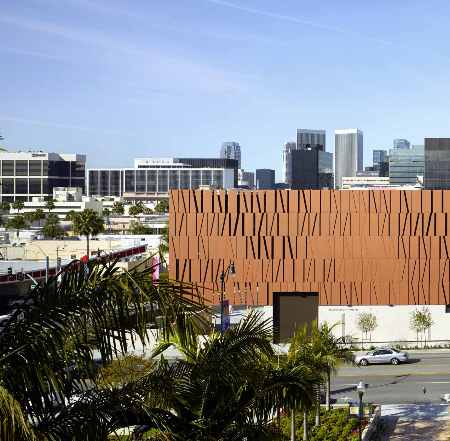
A skin of copper-toned Swisspearl panels in the shape of different letters envelops the new theater building, referencing the former use of the site as a post office.
